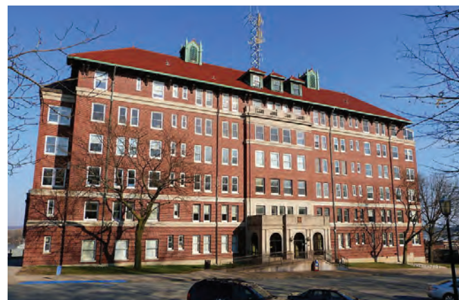
Mercy Hospital, only remaining building
